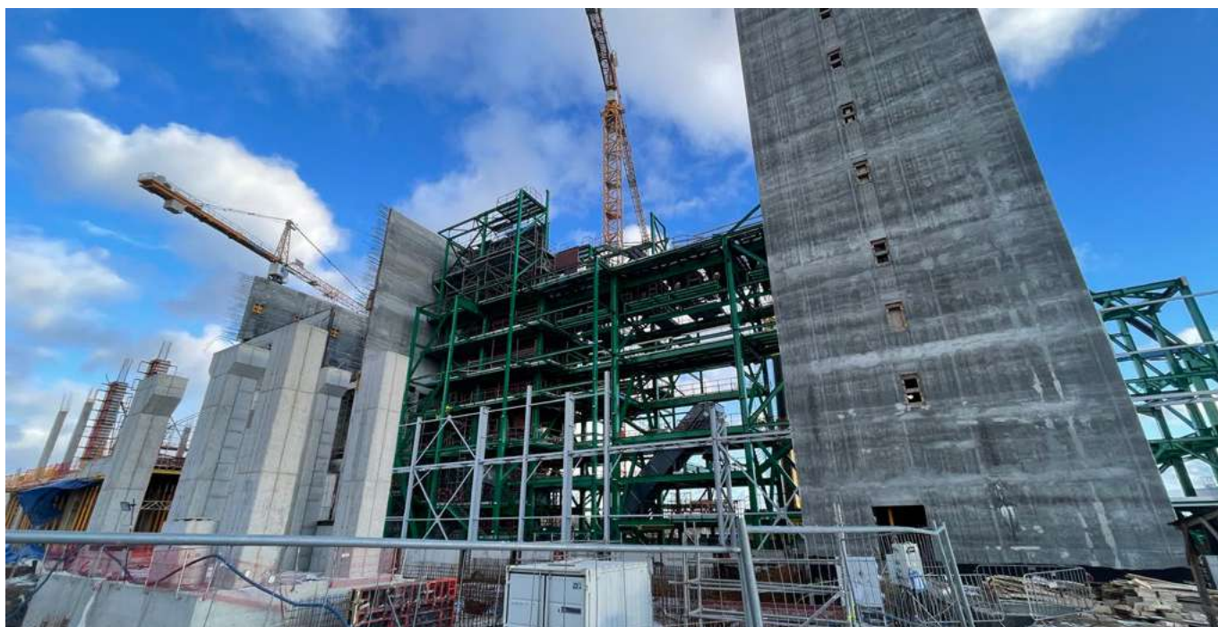
Construction of a WTT in Olsztyn
