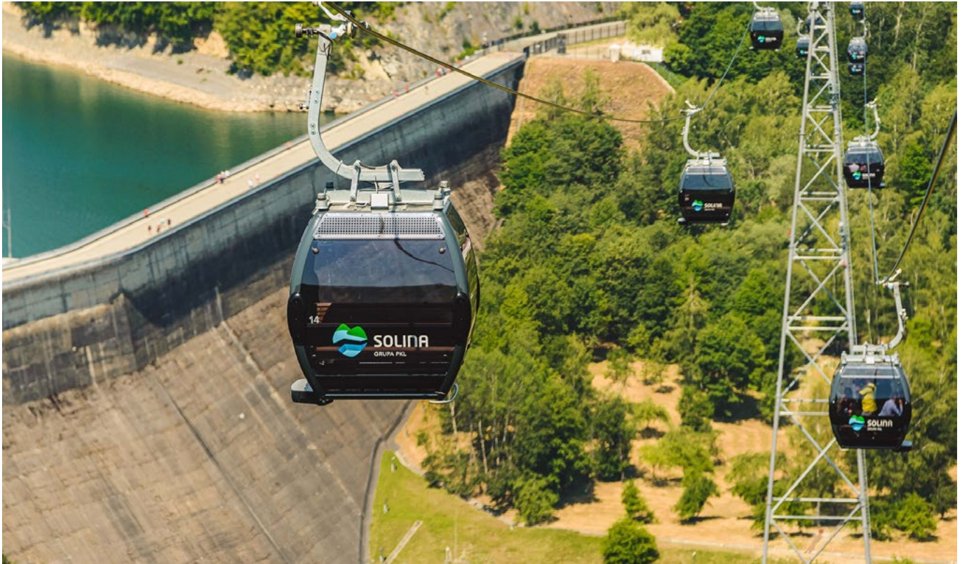
Cable car line over the Solina dam
