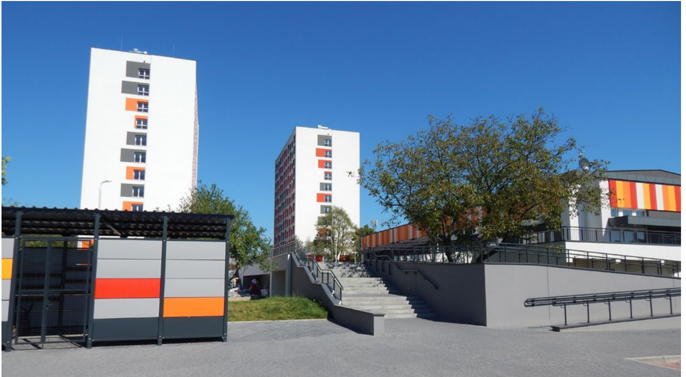
Student dormitories at ul. Badurskiego in Kraków
