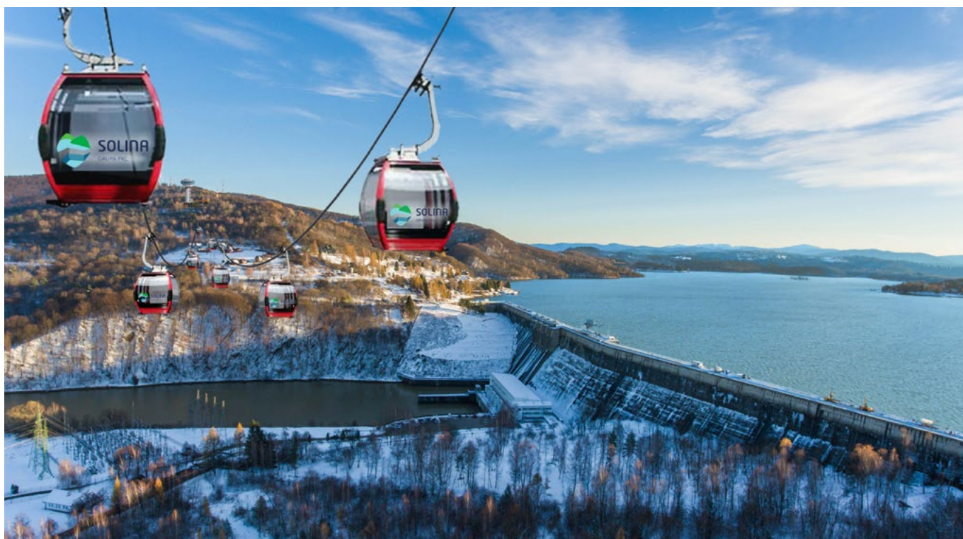
Cable car line project over the Solina dam in Bieszczady
