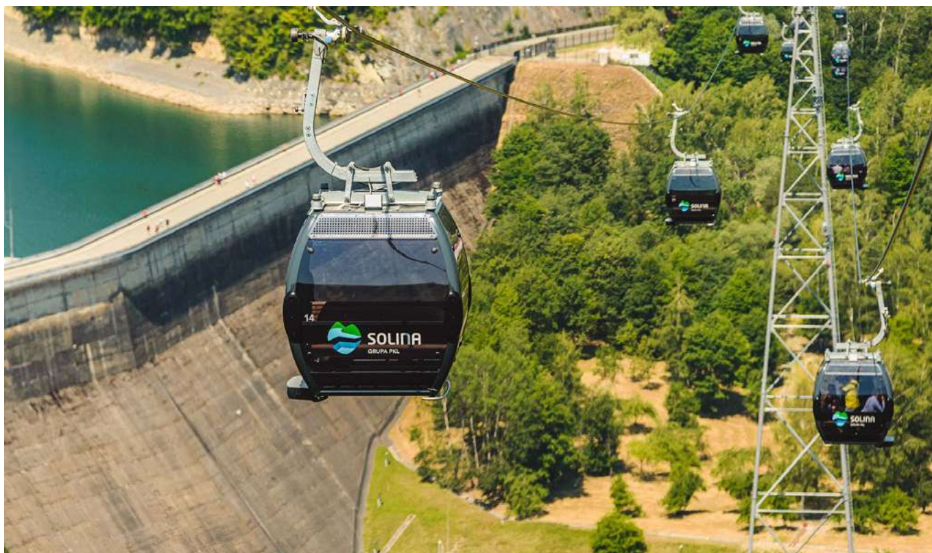
Cable car line over the Solina dam
